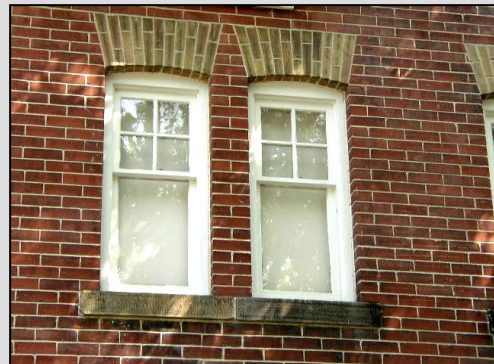
All the front windows on the second floor have single-hung divided sashes, which means they have smaller upper sashes with four panes each, and larger lower sashes with a single pane.
