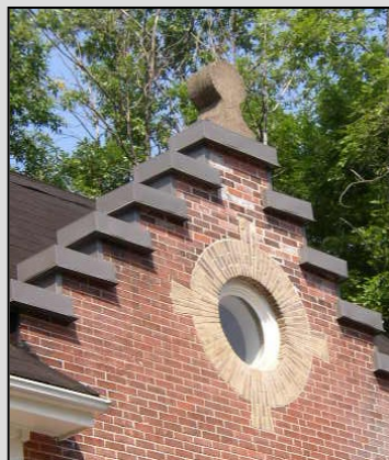
Buff brick, with brick "Dart" at the quarters of the circle surround the side gable. Only four buildings in Niagara-on-the-Lake have the use of buff brick for decoration around openings.
