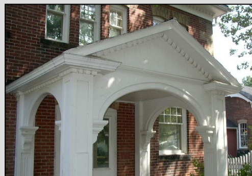
The columns on the porch are spanned by a corbelled arch.
